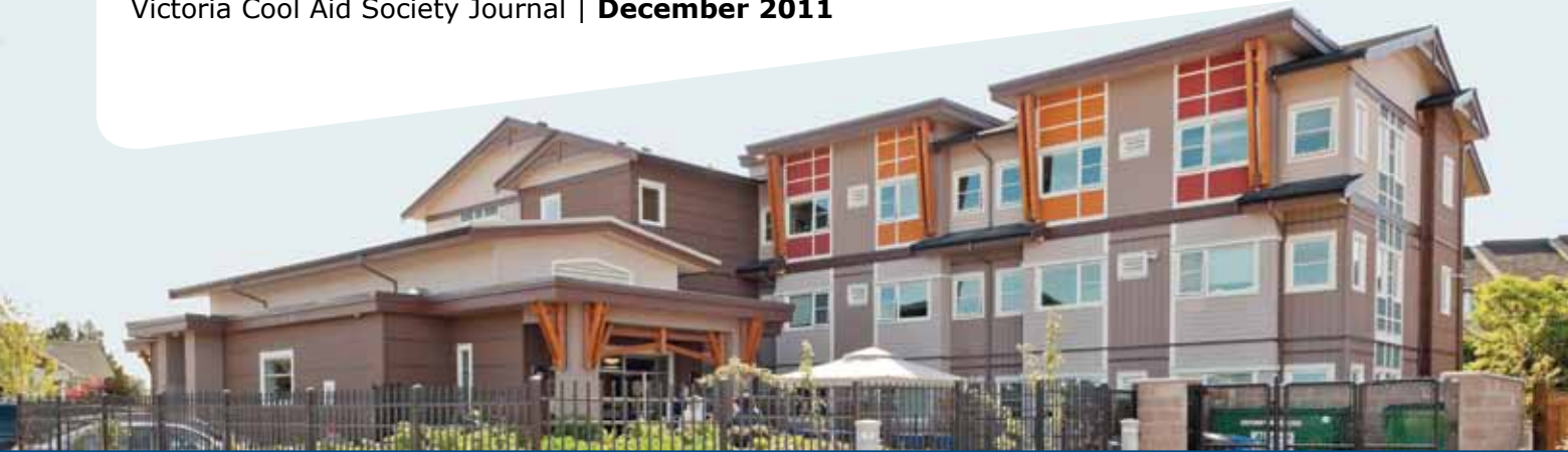
Olympic Vista seniors housing in Saanich is one of two new housing buildings opened this year; the other is Queens Manor, an old Travellers Inn.
